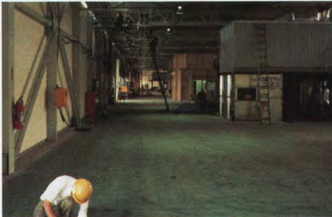
The new plant at Sanage where its speedy construction took our Team completely by surprise. It is now complete and the official opening ceremony took place at the end of August.
